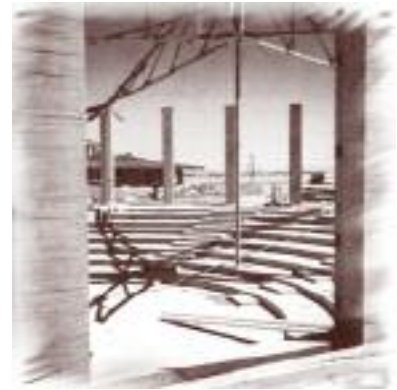
Cochise College under construction
